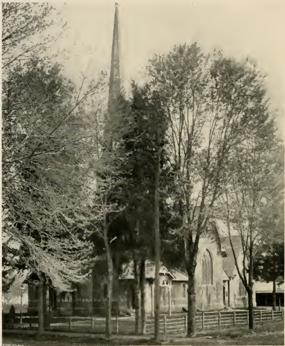
THE SCOTCH PLAINS BAPTIST CHURCH. ERECTED 1870.
